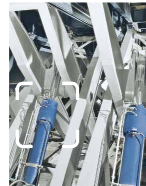
Elevating podium in the theater Stepless holding of the podium position
